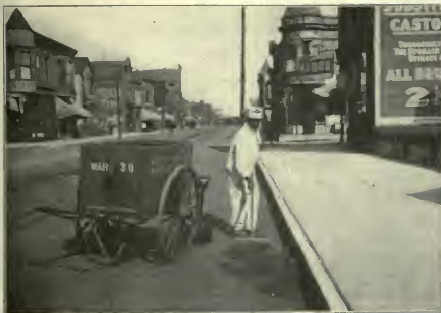
FIG. 60. STREET CLEANING OPERATIONS, A SOURCE OF DUST. Photograph taken September 1, 1914. Street cleaning as practiced in Chicago constitutes an objectionable source of dust.
